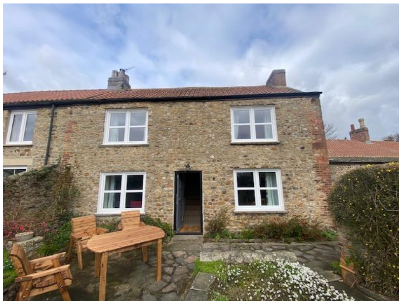
Rear access to the property
